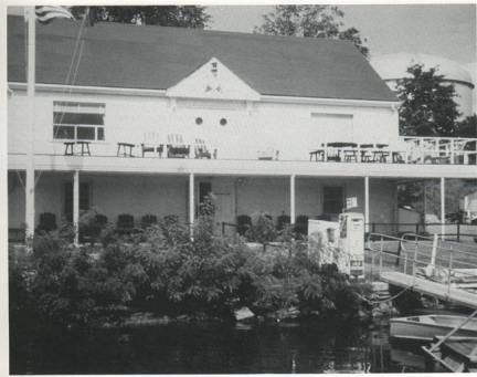
Clubhouse with new porch over the lower deck.
