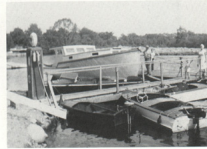
Original gas dock.
