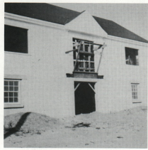
Early stage of construction of The Club House.
